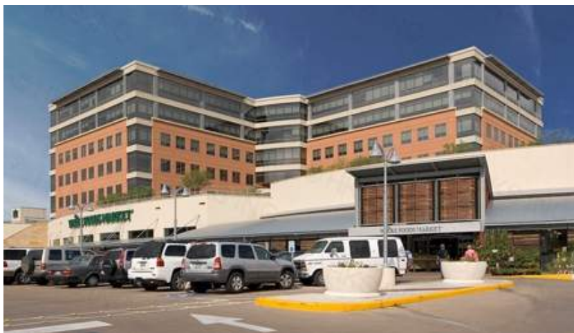
Retail Center, Parking Garage & Office Tower
