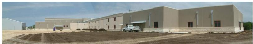
Exterior cladding consists of painted tilt-up panels and masonry veneer.
