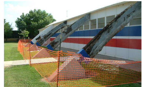
Prior to repair
