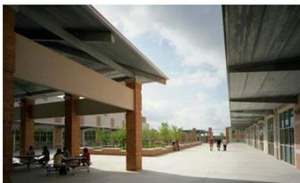
The buildings were provided with canopies cantilevered from the face of the tilt-up panels. Framing for the canopies and the breezeway covers consisted of galvanized tee beams, with the breezeway roofing supported by cast-in-place concrete columns. A pavilion, consisting of galvanized steel trusses with tubular steel rafters was provided, as a gathering area, between the fine arts and athletics buildings.
