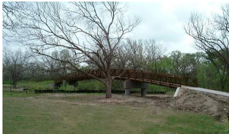
The bridge at hole #7 is 8 feet wide.
